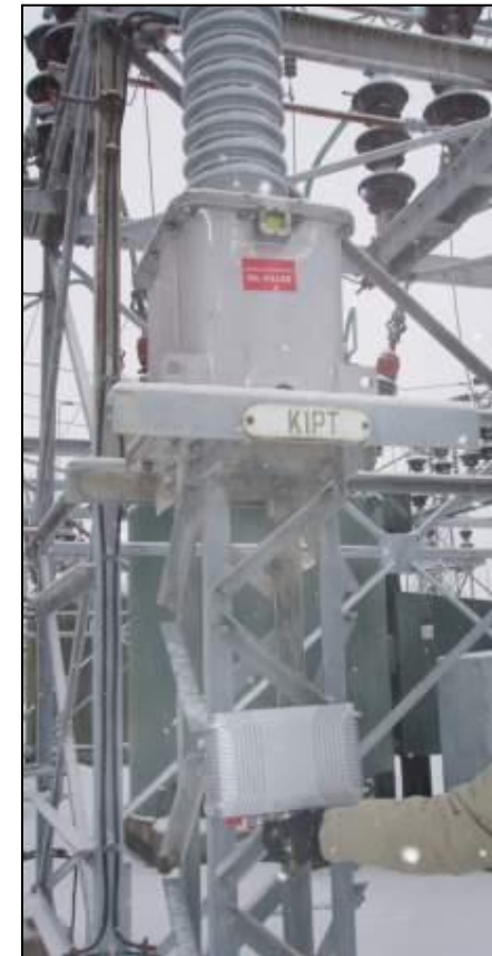
External, on a structure
